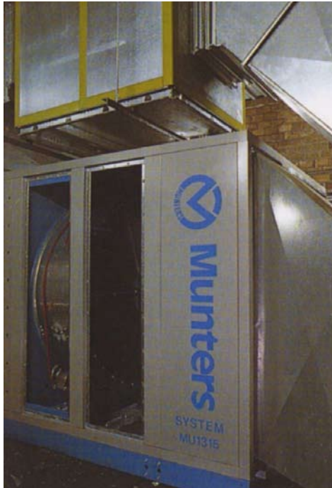
Advanced Munters dehumidification systems create safe working conditions.
