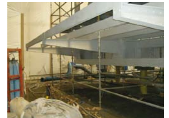
(1) A new bridge is being painted in the workshop before transportation. An enclosure protects the fresh paint from the environment and a dehumidifier regulates the climate.
