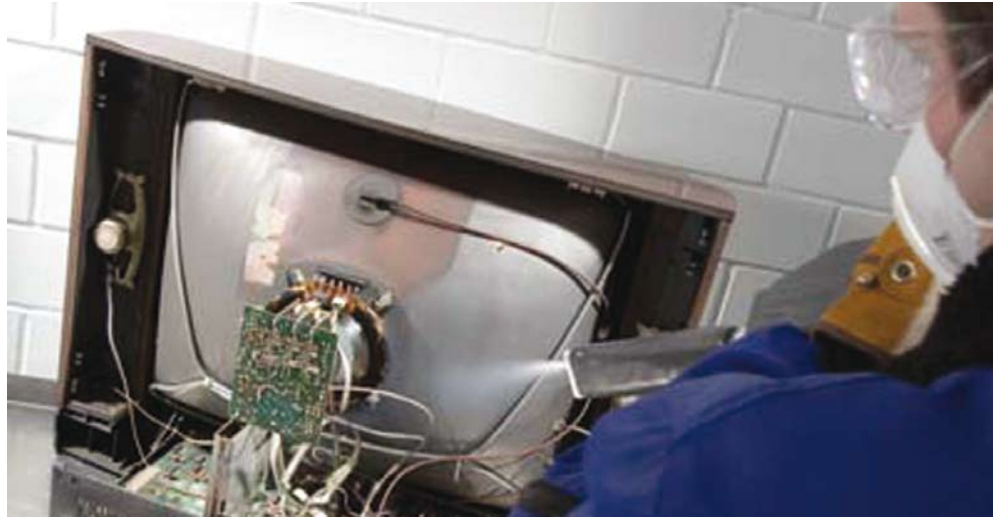
Dry ice blasting television circuit board.
