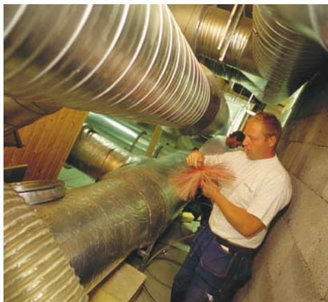
Cleaning using nylon brushes.
