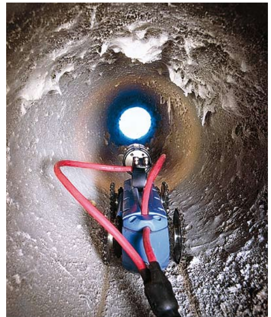
Inspection prior to cleaning using camera equipment.
