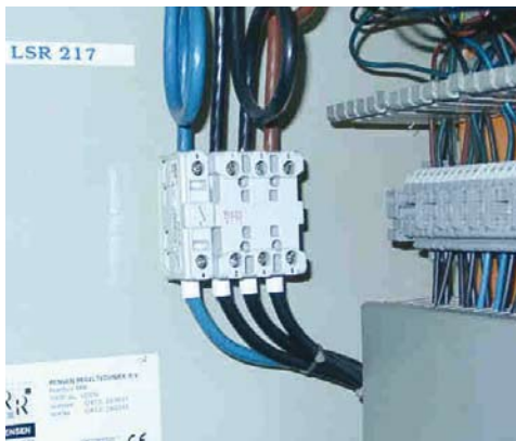
Non-destructive, thermography enables more efficient repairs.
